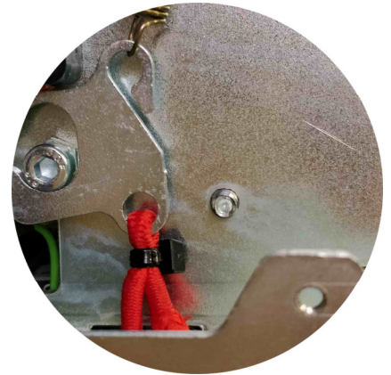
Figure 26, Replacing emergency stop cord.
